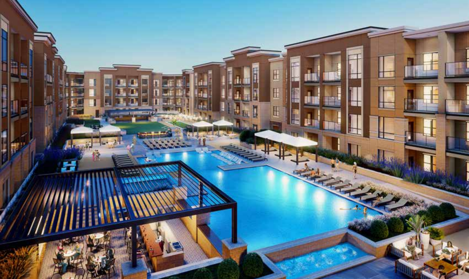
The Residences at Galleria is the first of two apartment communities planned at the Galleria mixed-use project located southwest of 112th Street and Nall Avenue in Overland Park, Kansas. The 322-unit apartment community broke ground in 2020 and sits on 5.74 acres. Once completed it will feature luxury amenities including a large resort style swimming pool, outdoor group fitness areas, cabanas, grill stations, and a host of other amenities.
