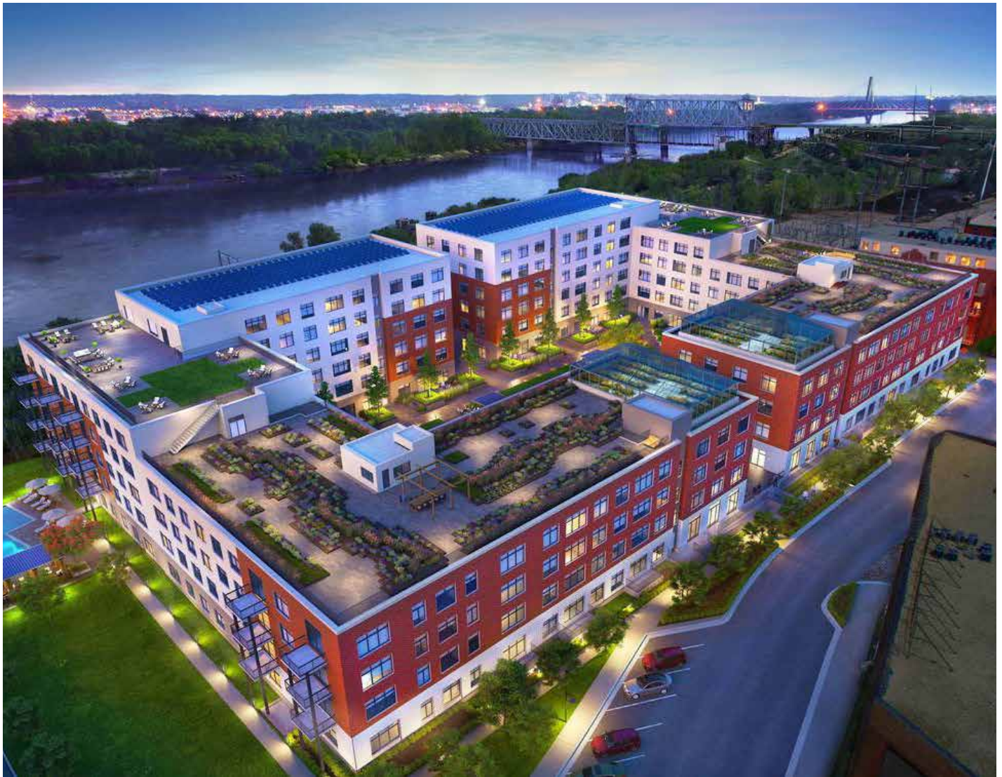
Touted as the world's largest structure to achieve Passive House energy-efficiency standards, the Second and Delaware apartment community is slated to open fall 2020 after the project stalled in mid-2017. Developed by Arnold Development Group the $96 million project will offer 276 units in the Kansas City River Market.
