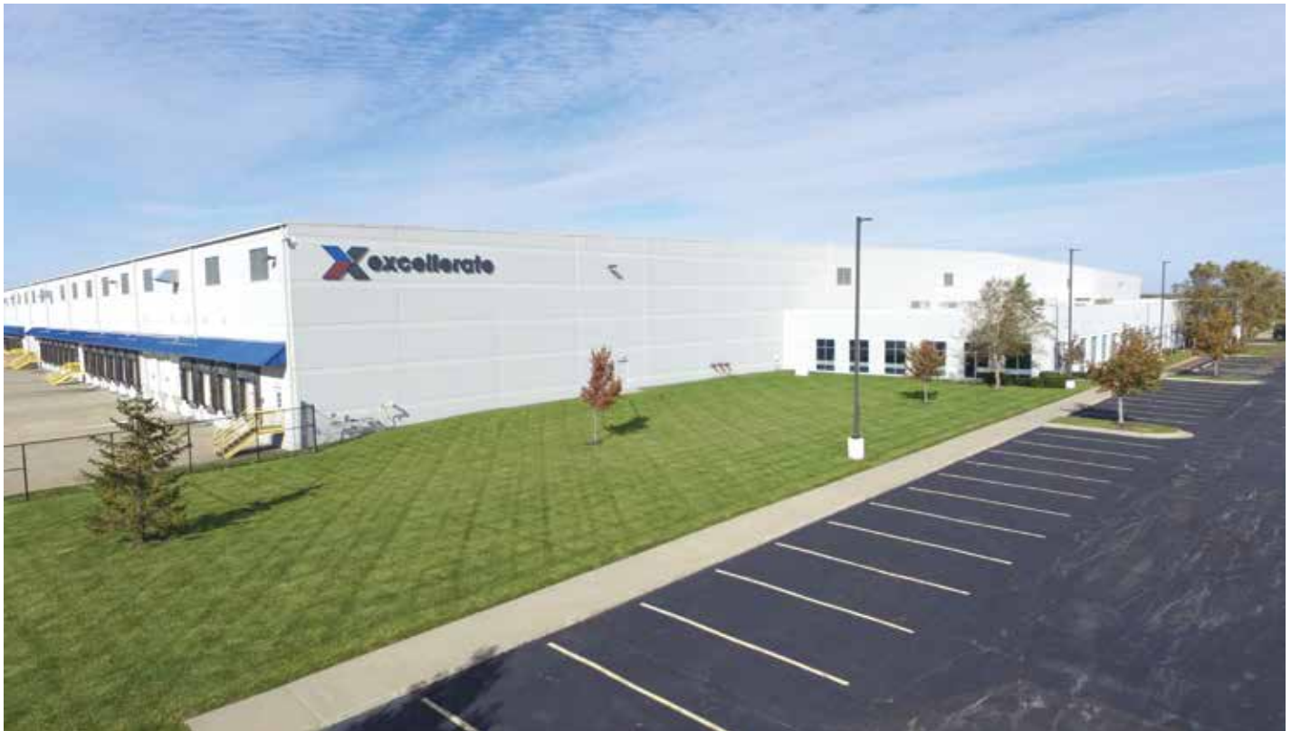
Faith Technologies, Inc. purchased the former PacSun Distribution Center for $20.8 million in July 2019. The 448,479 square foot industrial building located at 21800 W 167th Street, Olathe, Kansas was sold by a BRES sponsored investment group. Faith Technologies, Inc. will house two of their company divisions at the new location, Xcellerate Manufacturing and Faith Technologies University.
