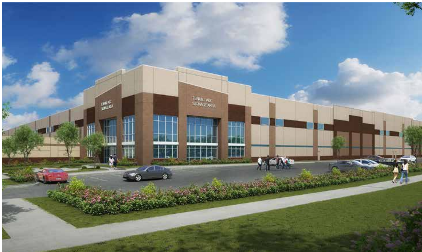
Construction began on Lenexa Logistics Centre North, the new 80-acre, $82-million industrial park northwest of College and Renner boulevards. The first of two 635,000 sq. foot industrial buildings is now under construction by BRES and is slated for year-end 2016 occupancy.
