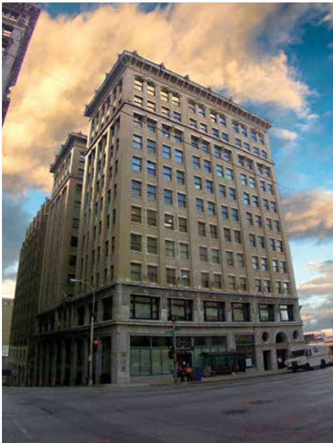
Developer Wayne Reeder acquired the 158,000 sq. foot, 12-story Scarritt Building located at 818 Grand Blvd. The developer plans to convert the building into offices with a 10,000 sq. foot event space.
