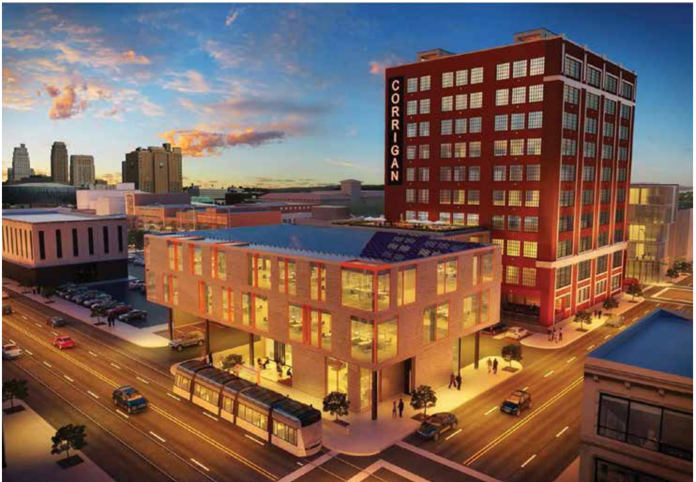
Copaken Brooks recently partnered with an investor group led by developer Vince Bryant on the $40-million project to transform the 10-story Corrigan Building into new offices. Originally, the 144,000 square foot building was set to be redeveloped into luxury apartments.
