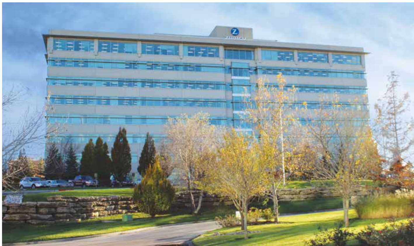
The Renaissance III building at 7045 College Blvd in Overland Park was purchased for $42 million at a 7.80% cap rate by St Paul Fire and Marine, a subsidiary of The Travelers Cos. Inc. The 233,820 square foot building is 100 percent occupied by Zurich American Insurance Co. and Intouch Solutions Inc.
