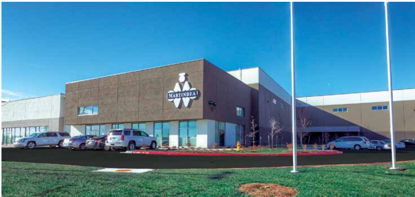
In 2015, a BRES-sponsored investment group acquired the Martinrea building in Riverside, Missouri for $19,950,000. The 369,000 square-foot property is leased to Martinrea International, Inc. on a long-term lease.
