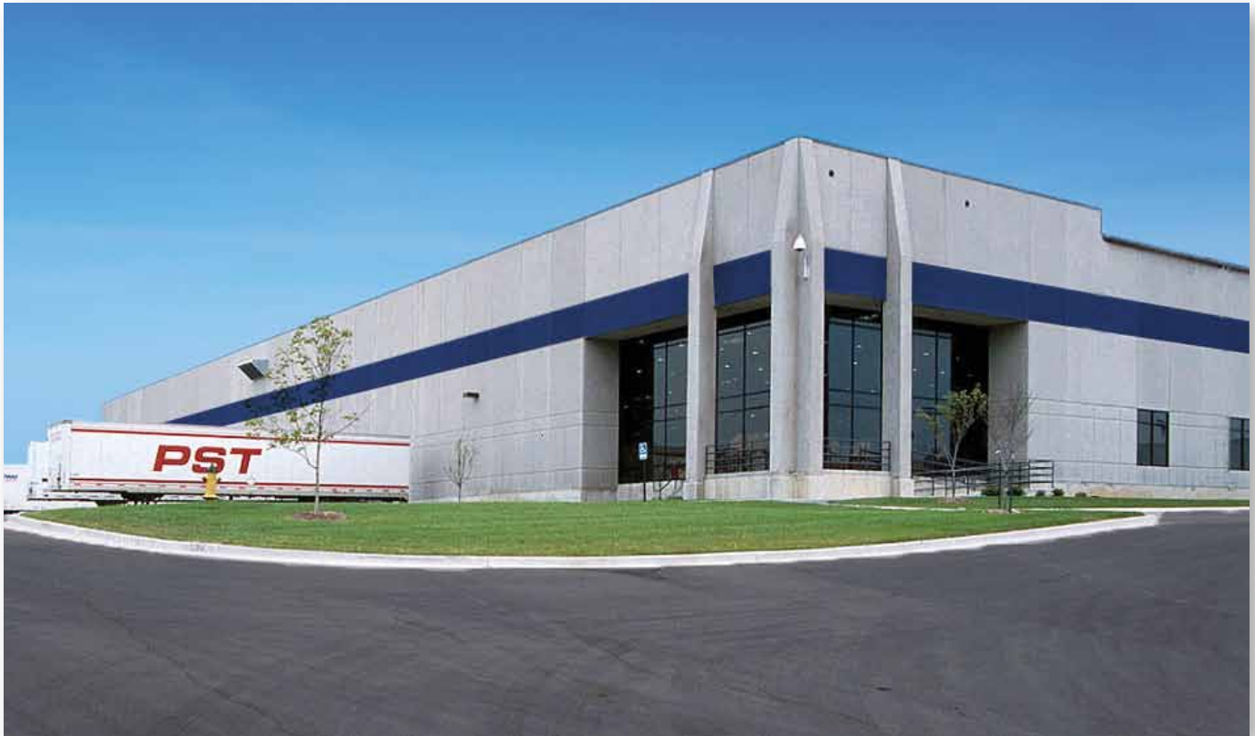
A BRES sponsored investment group acquired the 239,000 sq. foot, multitenant warehouse building at 16910-17000 W. 116th Street from Silpada Designs in September, 2013 for $10.4 million.
