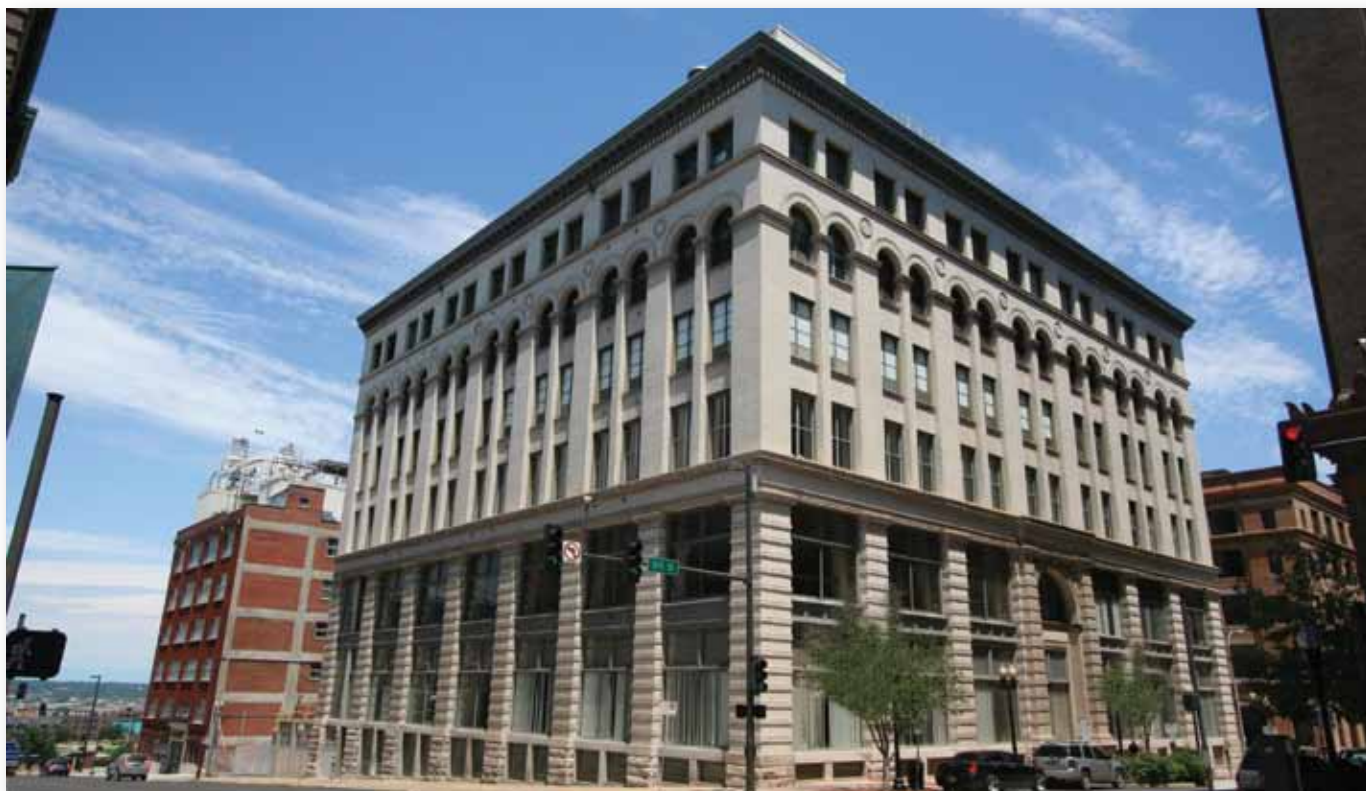
The six-story, 217,160 sq. foot Folgers plant closed and has been purchased by O'Reilly Development Company LLC of Springfield, Missouri with plans to redevelop the space into approximately 147 luxury apartments.
