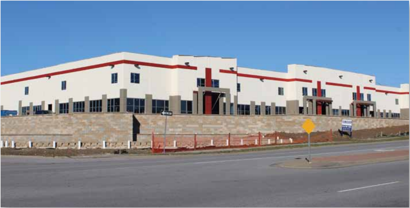
Block Construction Services nears completion on College Crossing K, located at College Boulevard and I-35 in Lenexa, Kansas. The park is 99% occupied and with the completion of Building K, the park's total square footage will increase to 530,000.
