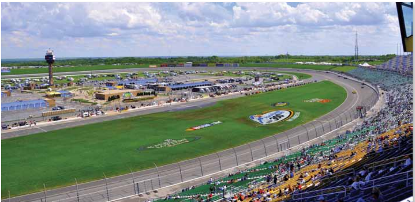
In 2012, the Kansas Speedway underwent a track reconfiguration and road course project, adding progressive banking and a road course in the infield. The speedway was built in 2001 and currently hosts two annual NASCAR race weekends.
