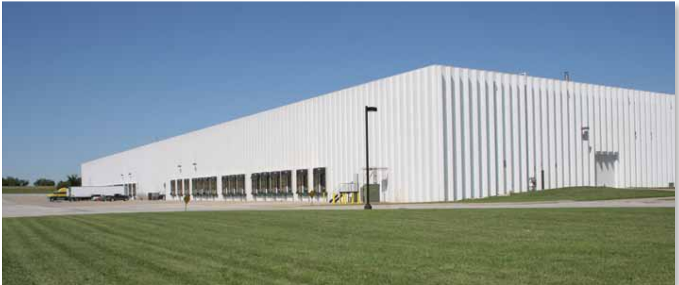
Botts Road Distribution Center, a 500,000 sq. foot facility in Grandview, Missouri, was purchased by a group of Block Real Estate Services investors, led by Managing Principal Ken Block. The building is fully leased to tenants Caravan Ingredients Inc. and Church & Dwight Co. Inc.
