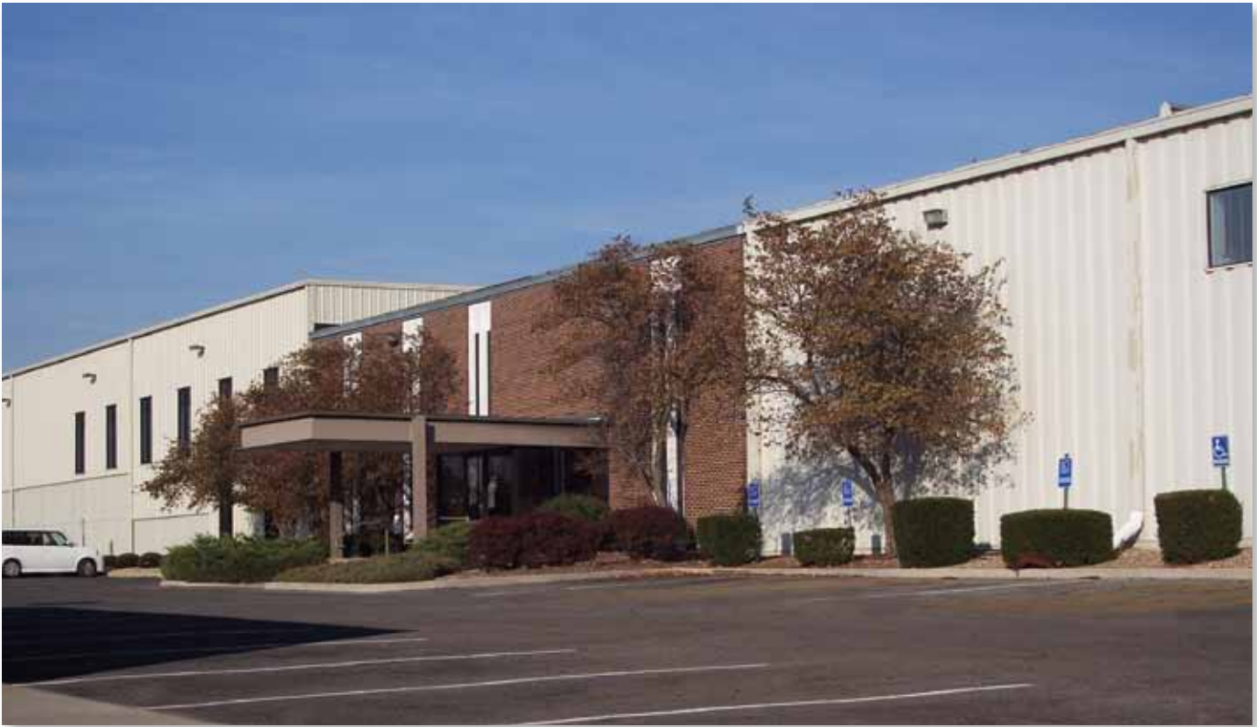
Quidsi Logistics LLC leased 100,940 square feet at 14601 W. 99th Street, Lenexa, Kansas, owned by a BRES sponsored investment group. The company also leased the entire 300,838 sq. foot industrial building at 11011 Lackman Road in Lenexa, and moved in to the space in June 2012.
