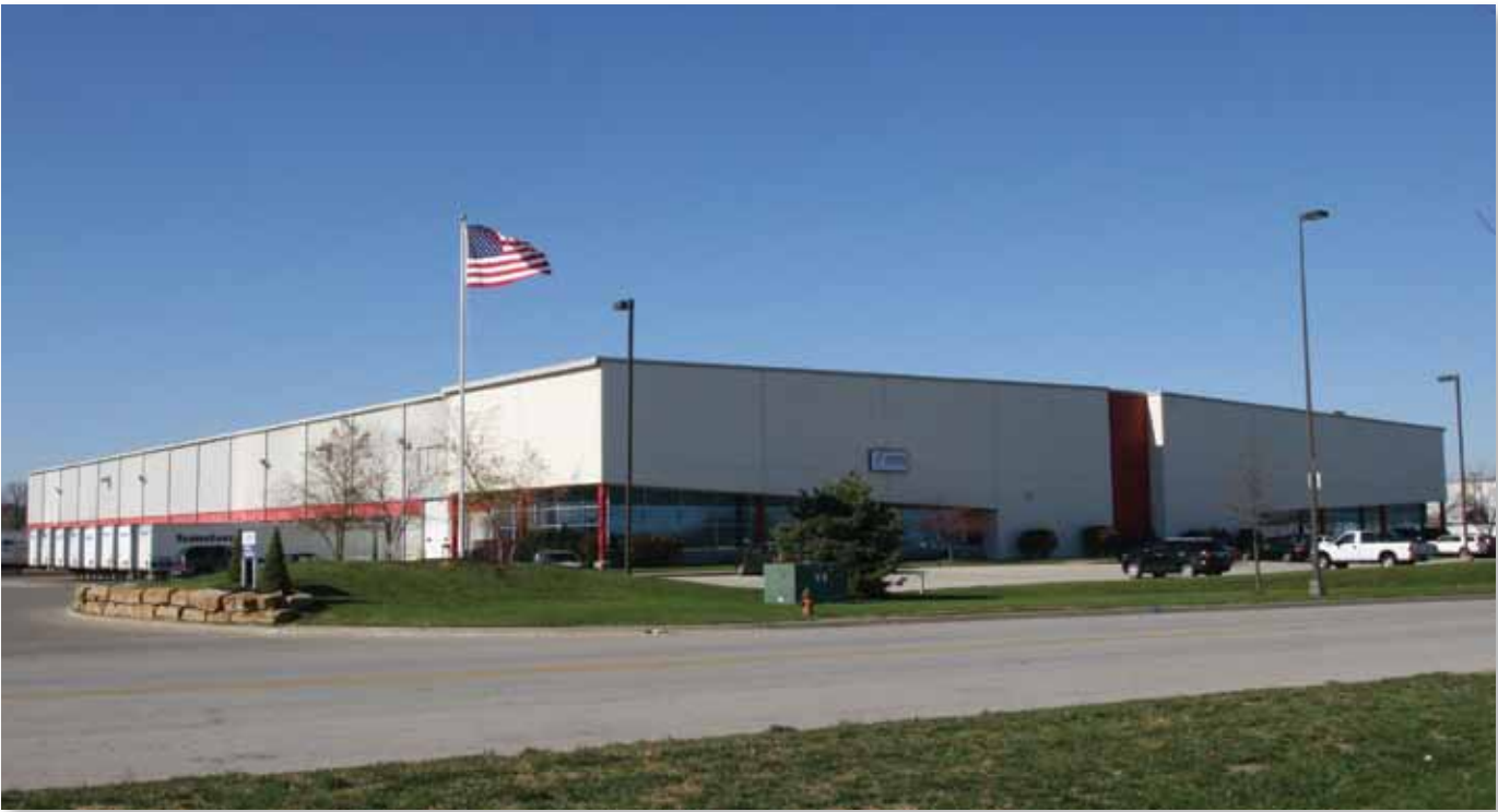
Heartland Sheets, LLC remodeled a 127,600 sq. foot building at 3950 N. Kimball Drive in the Northland Industrial Park, Kansas City, Missouri. The project cost $23 million and brought 43 jobs to the new manufacturing facility in Kansas City.
