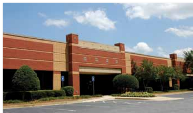
Siemens reached a lease renewal agreement for 56,000 square feet at our Lakeside building in Norcross, Georgia.
