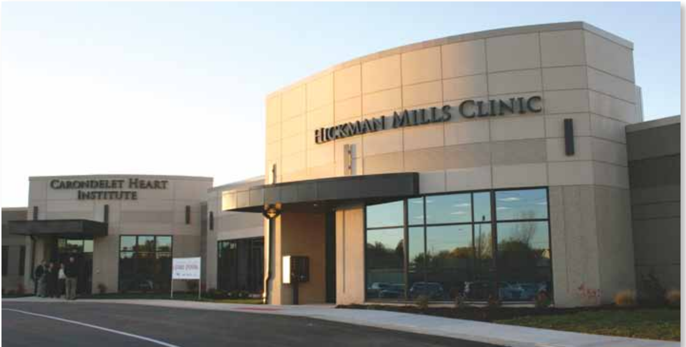
The 20,000 sq. foot Grandview Medical Building, home to Hickman Mills Clinic, Carondelet Heart Institute and Albers Medical Pharmacy, brings a high level of integrated outpatient health services to the Grandview, Missouri community. This project was developed by Block Healthcare and syndicated with some of the existing doctors and BRES investors.
